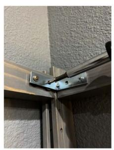
Attach "L" bracket to frame using 3/4" screws and plastic washers between bracket and wood.
